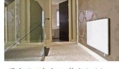
The heating technology used by Logicor in its systems is based on far infrared energy, which uses pulsed and phased electricity controlled by algorithms to make it extremely energy efficient. It doesn't heat the air but gives off infrared energy that heats the structure, furnishings and people within.
